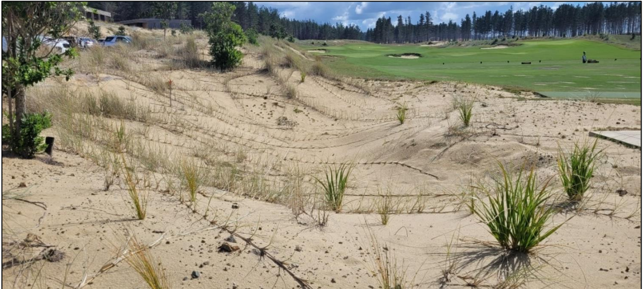
Photograph 4: Recently planted infiltration basing serving the overflow clubhouse parking, April 2023.
