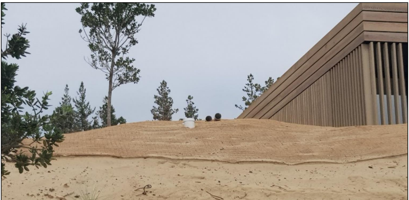
Photograph 5: Coconut matting used to stabilise dunes, March 2022.
