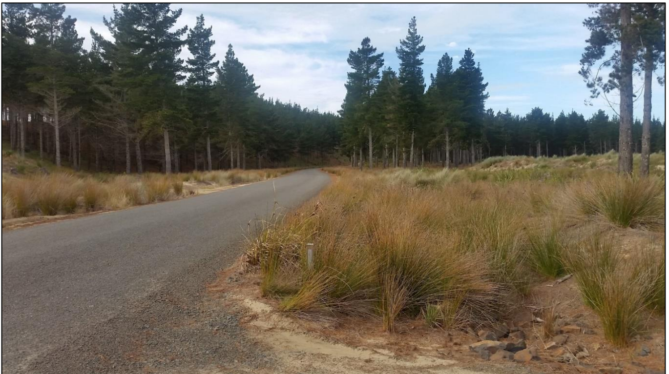
Photograph 3: Fully planted vegetated swale.
