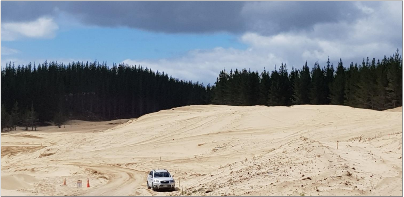
Photograph 2: Typical sandy soils during golf course construction, November 2020.
