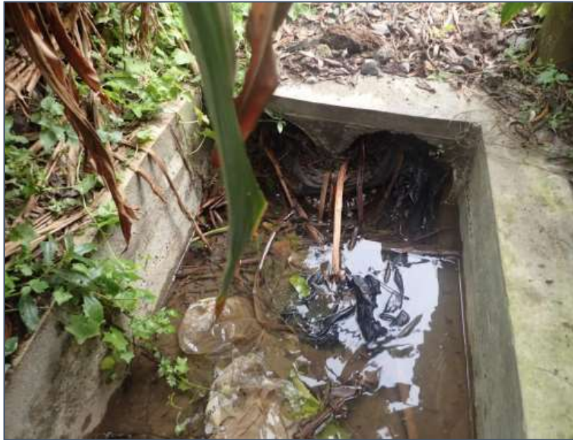
Photograph 1: Auckland stormwater inlet to a portion of a piped, unnamed stream.
