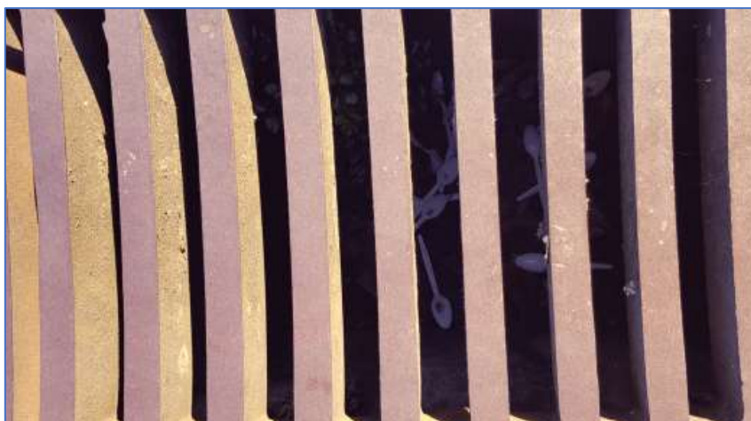
Photograph 2-4: Catchpits with macro plastic present.
